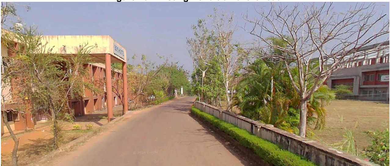
Figure 10: Existing Condition of the road
