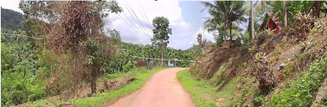
Figure 26: Existing Condition of the road
