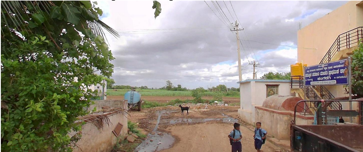
Figure 2: Existing Condition of the road
