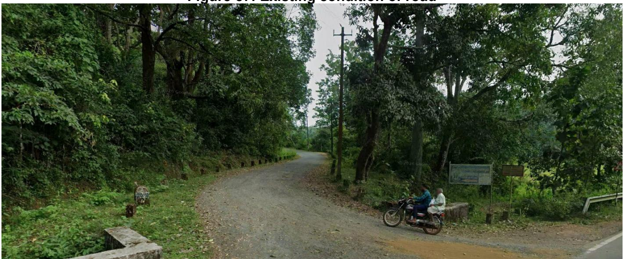
Figure 57: Existing condition of road
