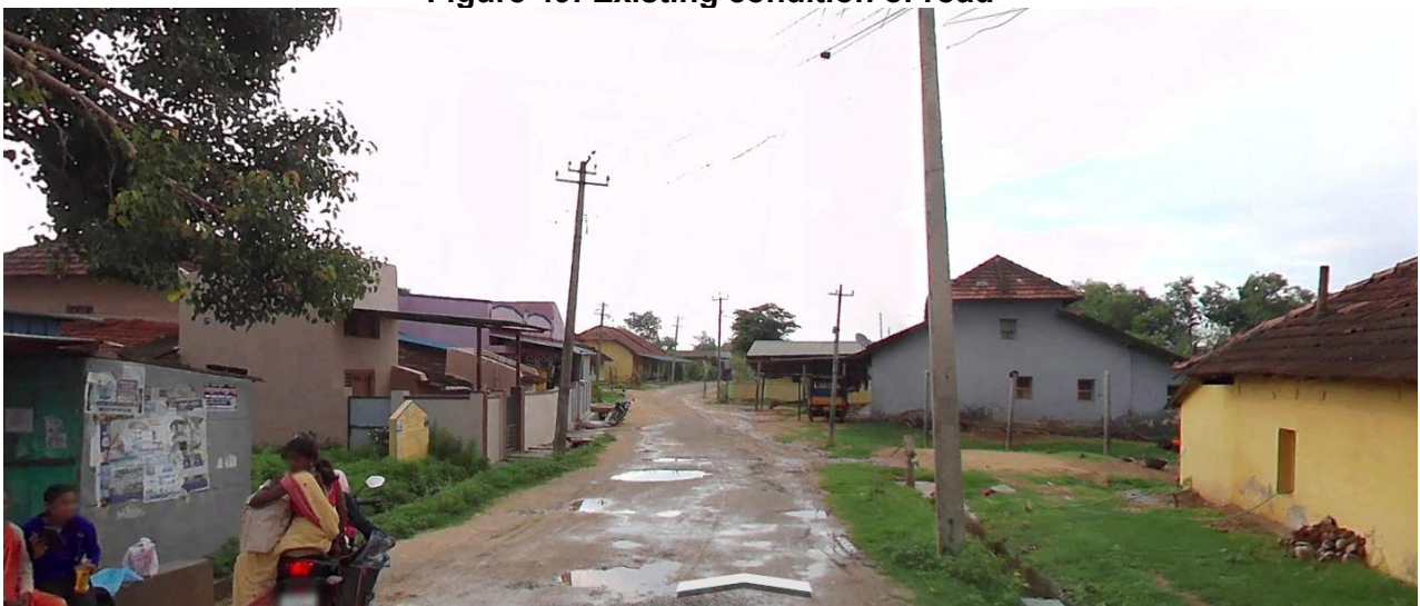
Figure 49: Existing condition of road
