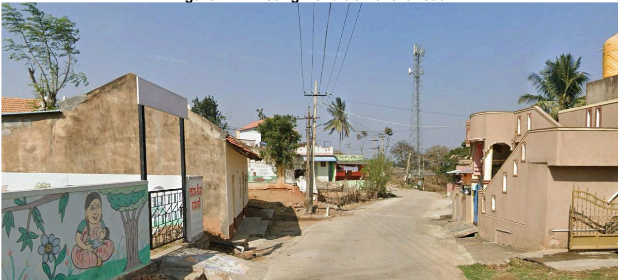
Figure 72: Existing Condition of the road
