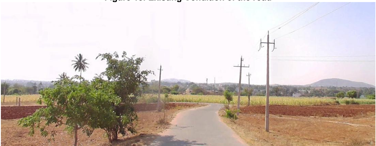
Figure 18: Existing Condition of the road
